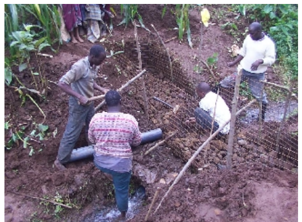
A wire mesh gabion filled with stones and clay
