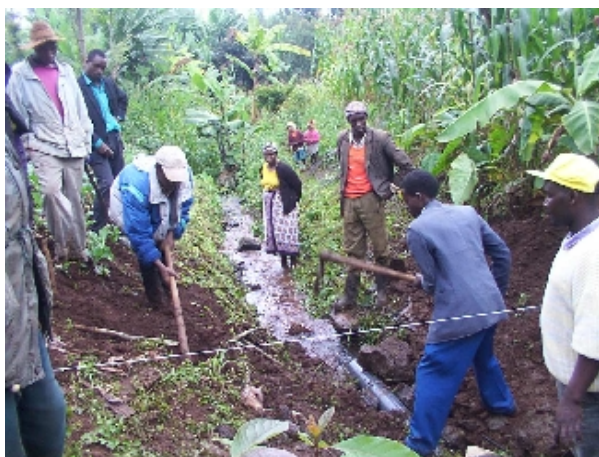
Preparing foundations for the weir
