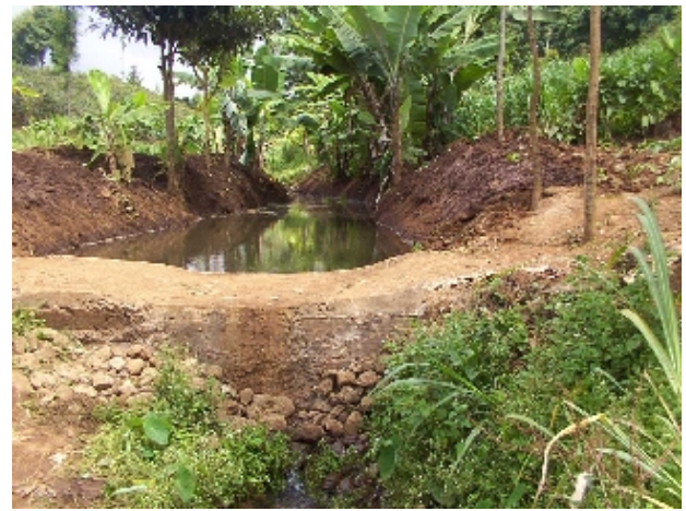
Completed intake with storage pond
